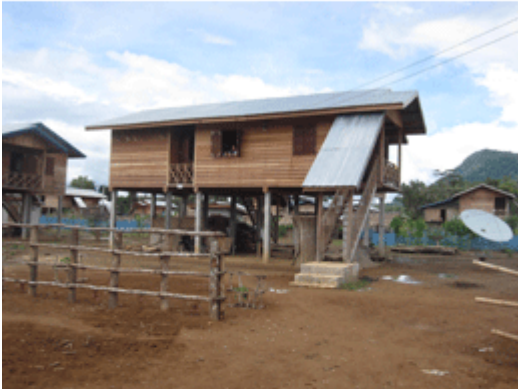
New housing being built in the Mekong region
