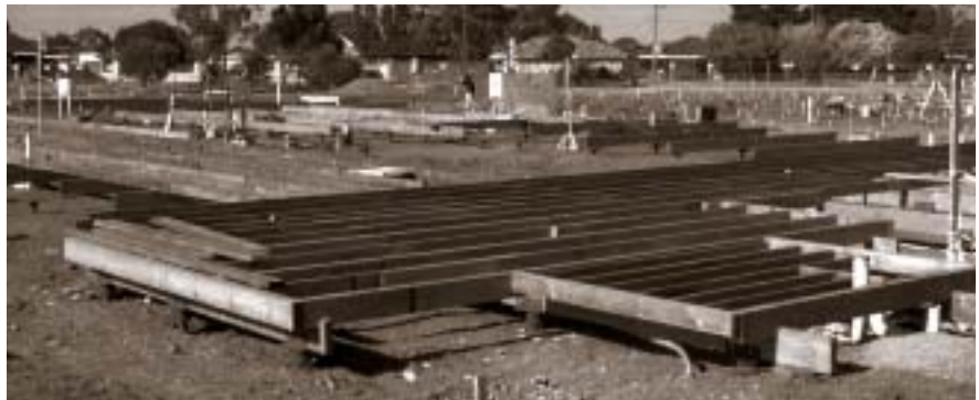
Construction of Alfred Felton House.
